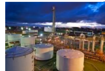
Refining Operations in Peru 1994-2015
